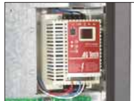
variable speed motor drive
